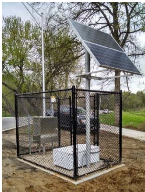
Figure 6 – Solar powered controls
