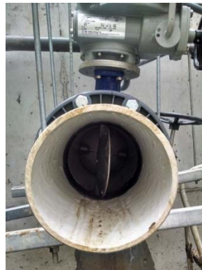
Figure 7 - Butterfly valve controls
