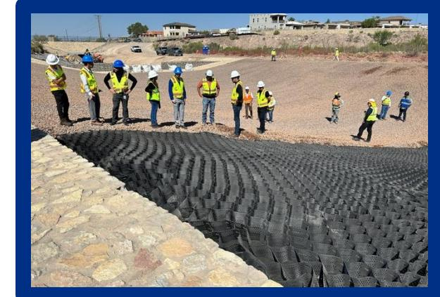
First EPWater project to utilize geogrids, a low-lying material that provides stability and prevents erosion.
