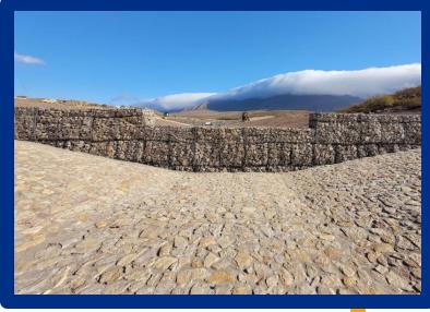
Gabion structures provide structural functions while blending into natural surroundings.
