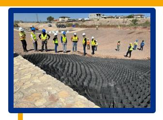
First EPWater project to utilize geogrids, a lowlying material that provides stability and prevents erosion.
